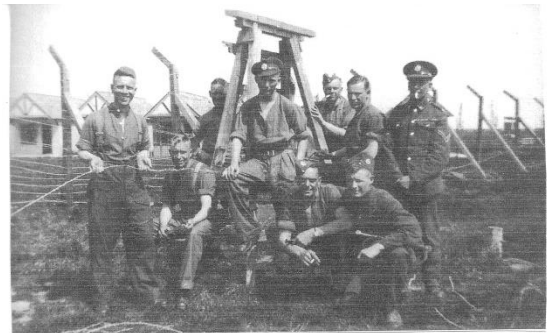
Warner's Holiday Camp 1940, Engineers from Harwich Garrison erect high protective fencing
