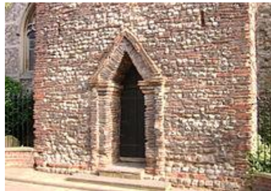
Saxon doorway of 11 th century Holy Trinity Church in Trinity Street. Colchester, reusing Roman materials
